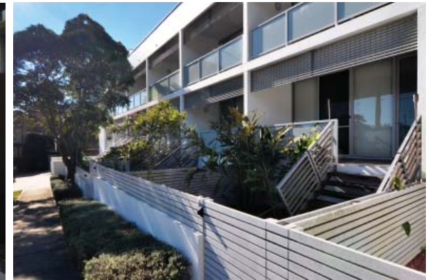
Figure 100: Step up from footpath to ground floor
